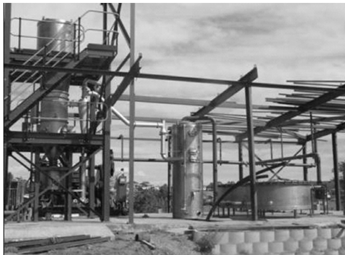
Fig. 1. The experimental gasifier installation at Melani village. The tall tower on the left is the reactor where gasification takes place, the low circular tank on the right is a sawdust filter, and the vertical tower in the centre of the picture is a gas scrubber.
